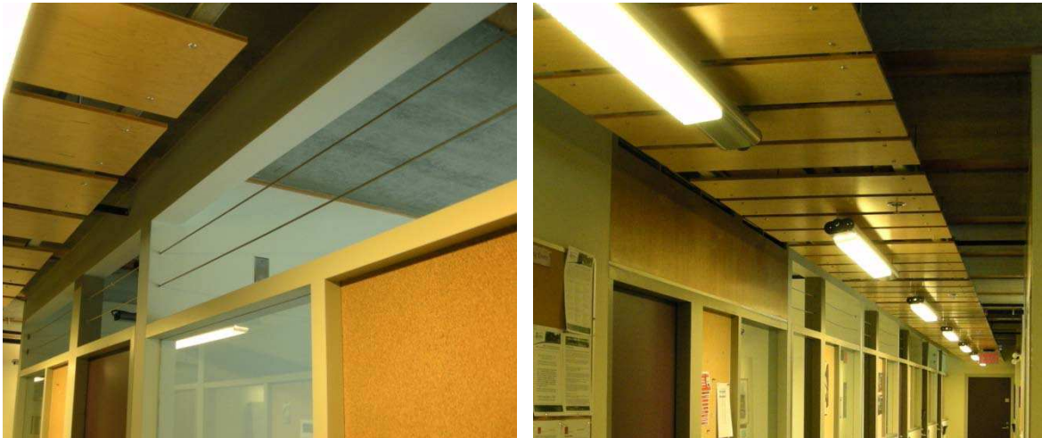
Figure 8. Gaps above doors in Building Q (left), and remedial measure for acoustic concerns (right).
